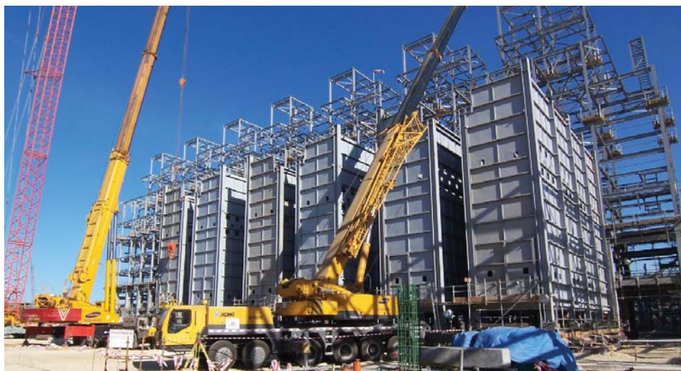
Construction services provided by Selas Fluid on an ethylene plant
